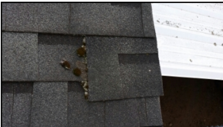
One roof shingle loose. Recommend having a roofer repair.
