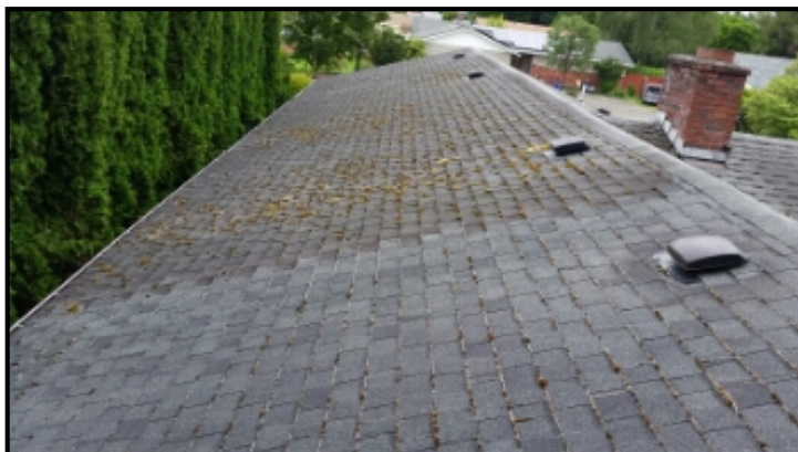
Maintenance Tip: Weather permitting, keep debris cleared from roof valleys to extend life of roof.
