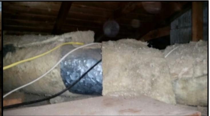
Warm air return found smushed. Recommend further review by an HVAC professional.
