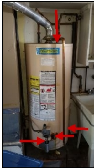
Gas heated water heater in garage. Recommend replacement. Leaks observed.
