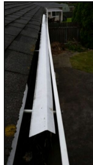
one or more areas where drip edge flashing has come loose. Recommend having a licensed roofer inspect and repair.
