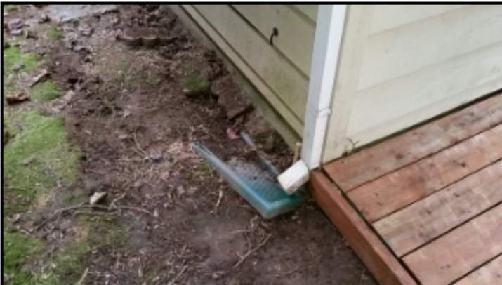
Extensions / Splash blocks missing or insufficient: Install to divert water away from the foundation.
