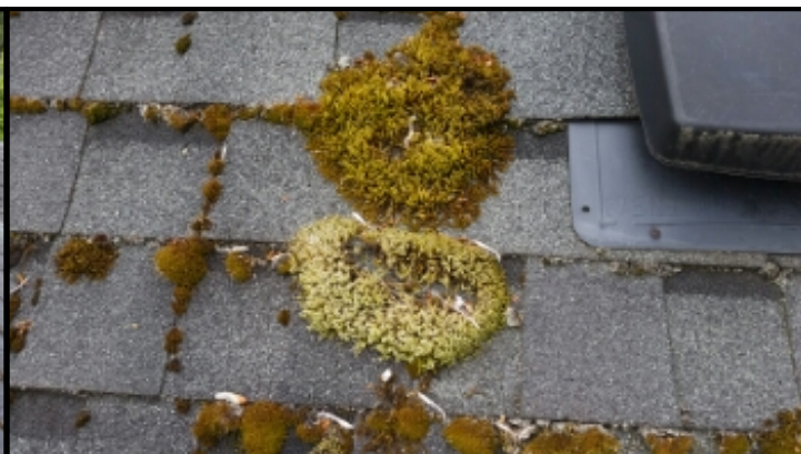
Moss on roof. This can lead to the premature failure of the roof and subsequent leaks. Recommend treating moss during its growing season (wet months) with a moss killer.
