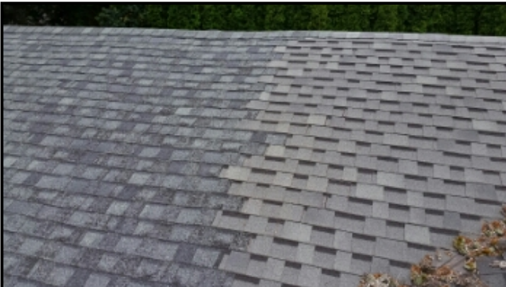
Sway in ridge beam is where the 2006 addition met the barge rafter. Appears to be done correctly.
