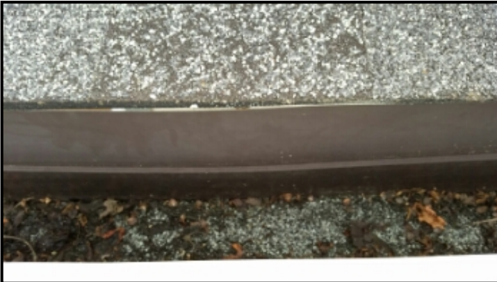
Gutter not under drip edge. possible opportunity for rafter tail dry rot. Recommend having them re-secured.
