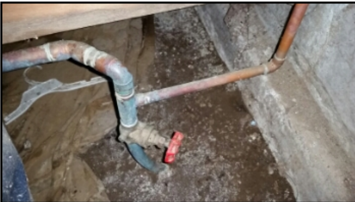
Main water shutoff found inside crawlspace access door in back closet.
