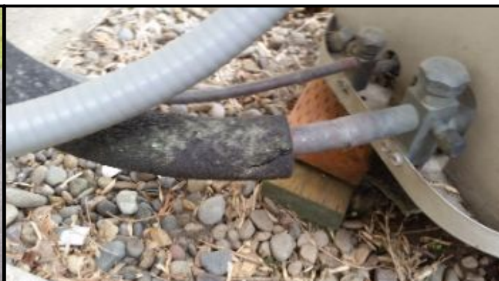
Condensate line (larger line) is not completely insulated. REcommend insulating to avoid rusting the exterior of the HVAC unit.
