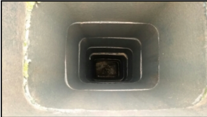
Terra cotta chimney liner. Chimney missing rain cap. Recommend installing chimney cap with spark arrestor to keep birds out and hot cinder off your roof.
