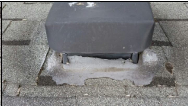
This roof vent appears to have been sealed post installation, but the sealant has failed. Recommend a licensed roofing contractor review further after it has rained.
