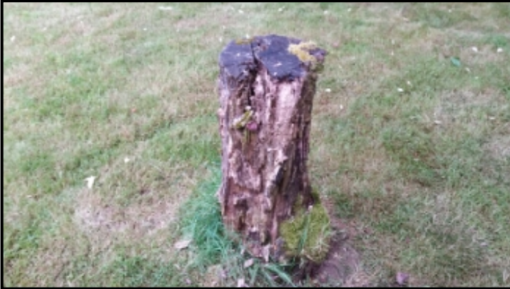
Stump in back yard may be hosting wood destroying organisms (WDO). recommend removal and treatment of soil by a professional exterminator
