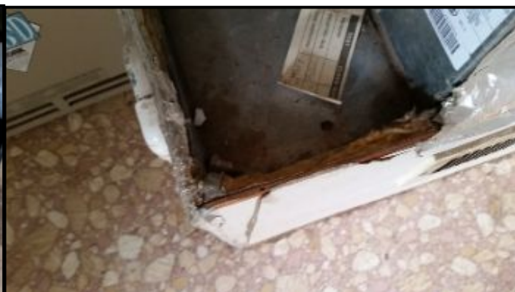
Bottom plenum at the furnace is made of wood. Recommend replacement by an HVAC professional.
