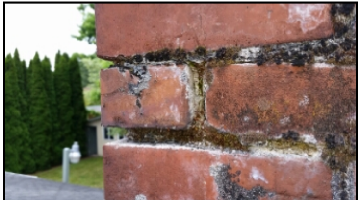
Chimney Mortar shows sign of deterioration. Recommend having repaired as necessary.
