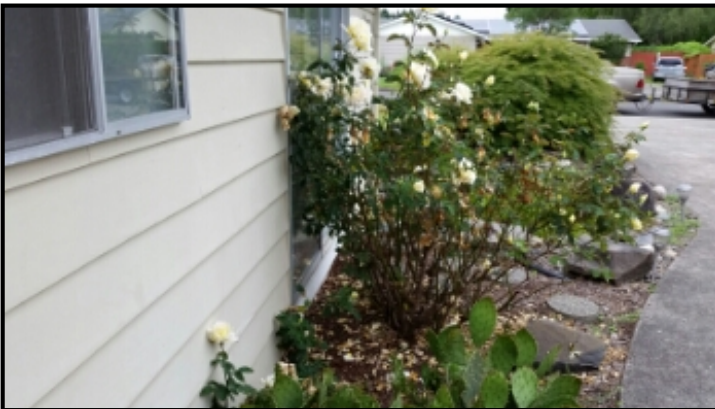
Vegetation in contact with siding which doesn't allow for siding to dry out after a rain. Recommend trimming or removal to leave a 12 inch gap between vegetation and siding.
