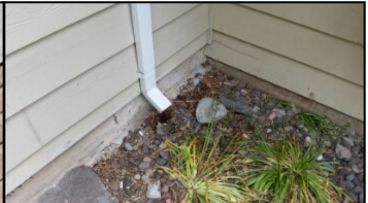
Extensions / Splash blocks missing or insufficient: Install to divert water away from the foundation.
