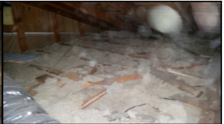
Insulation averages 3 to 4 inches. Recommend installing more.
