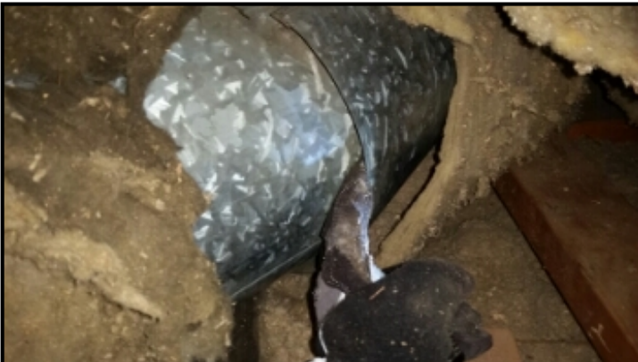
Warm Air return has sizable leaks. recommend having this inspected and repaired by an HVAC professional.
