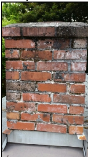
Chimney is made of brick and mortar.
