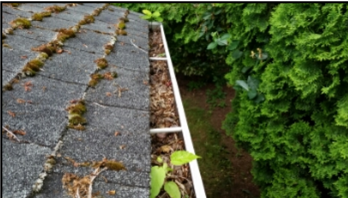
Gutters full of debris. Recommend removal of debris in order for water to channel towards the downspout.
