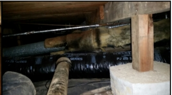
Soft duct laying on floor. Recommend suspending this duct from the floor joists for a longer lasting product.
