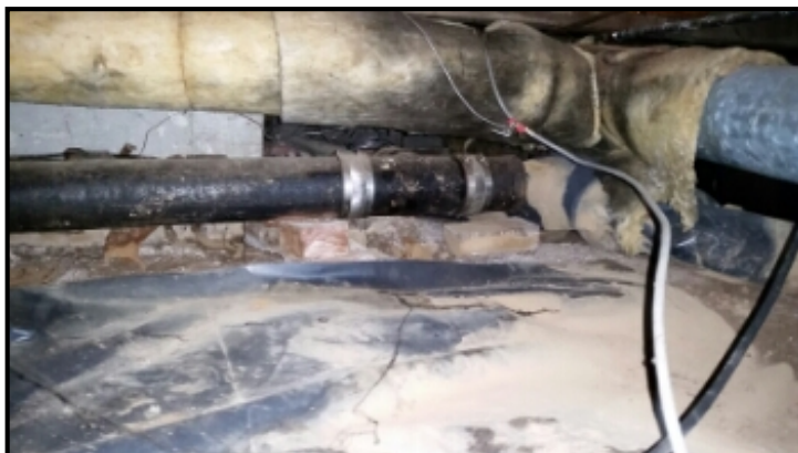
Signs of duct leakage. Recommend having your ducts tested and sealed.
