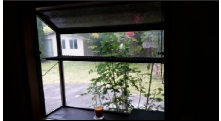
Duel glazed garden window in kitchen appears to have broken seals.
