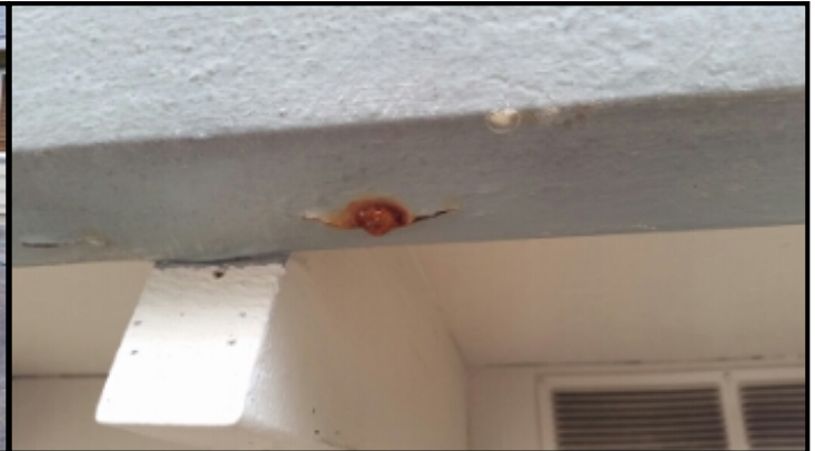
leak found in gutter above garage door
