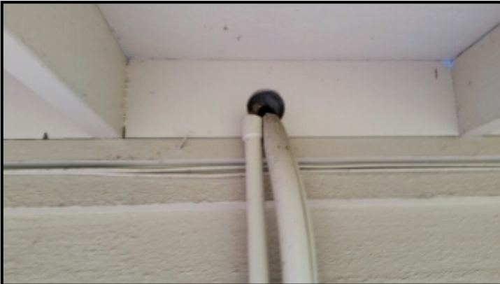
Air conditioner coolant and power access hole. Conduit stops short of hole and should be reviewed by electrician for possible wear on cable. Recommend sealing
