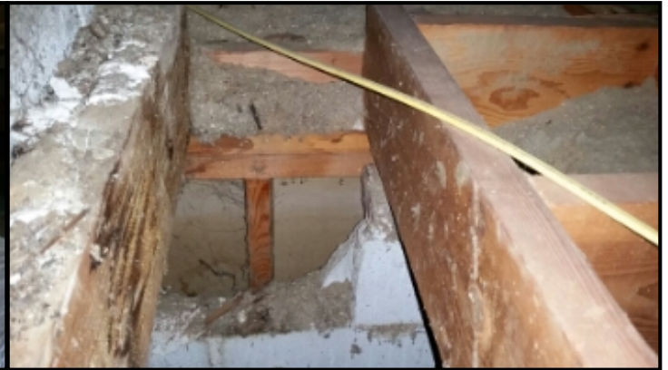
Brick and mortar missing at kitchen wall. recommend sealing to avoid heat loss.
