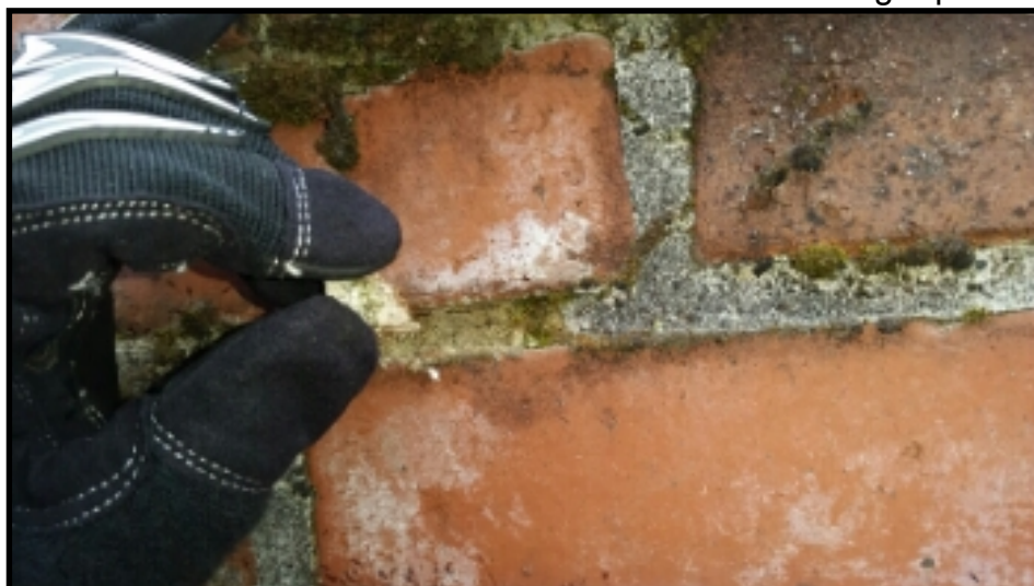
Chimney Mortar shows sign of deterioration. Recommend having repaired as necessary.
