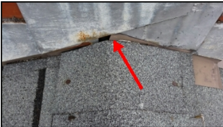
Questionable flashing at chimney. there appears to be a gap at the step flashing. Recommend having a licensed roofer inspect further after it has rained.
