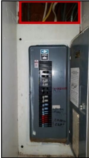
Zinsco service panel. Recommend removal due to age and inherent problems with materials used. panel screws missing. Unshielded wiring above panel.
