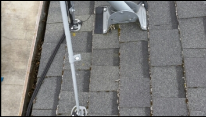
Satellite dish mounted on roof. Self Sealing membrane appears to have been used to avoid moisture penetration. Good Installtion.
