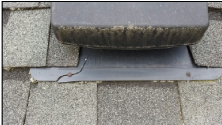
Roof vent(s) damaged. Recommend replacement by a licensed contractor.
