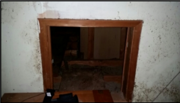
Access door to attic found open. This should be closed to slow the course of fire that may start in garage.
