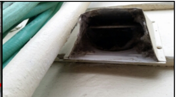
Dryer vent stuck open with lint. recommend cleaning so it can close and avoid pest intrusion.
