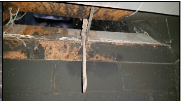
Damper hardware damaged. It is stuck in the open position. This is both an energy waste and an opening for pests. Recommend repair by licensed professional.
