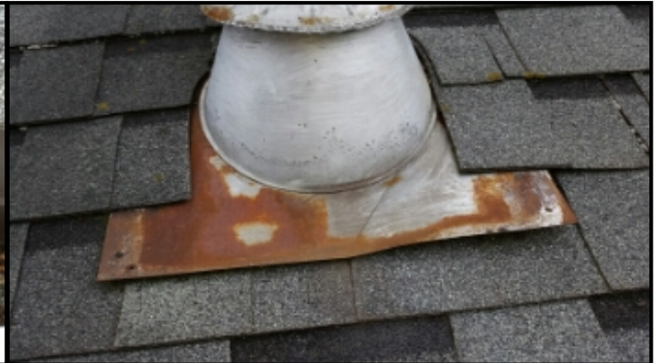
Apron flashing at roof vent peeling up. Recommend having a roofer inspect and repair if necessary.
