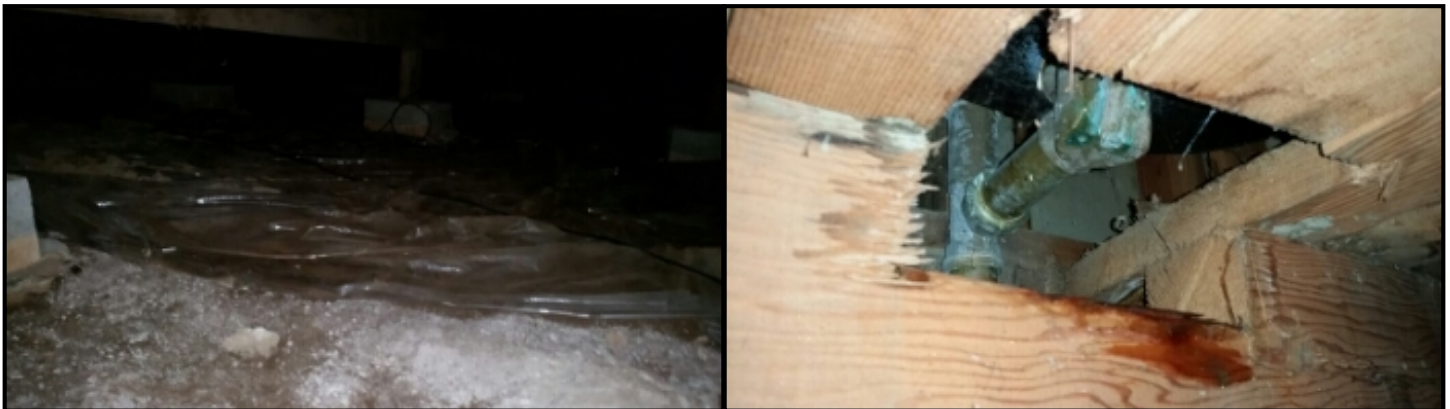
Vapor barrier incomplete. Recommend replacement
