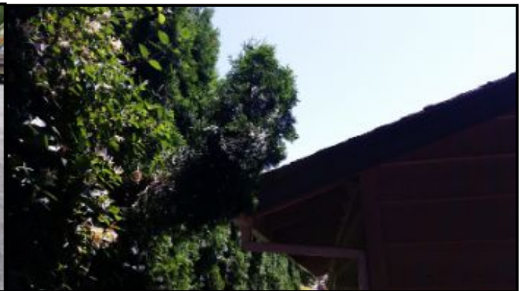
Arborvitae in contact with house. Recommend removal of limb.
