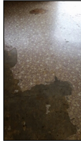
Minor settlement cracks in garage observed where linoleum had peeled up.
