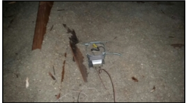
Open junction box in attic. Recommend having it covered by a professional electrician.
