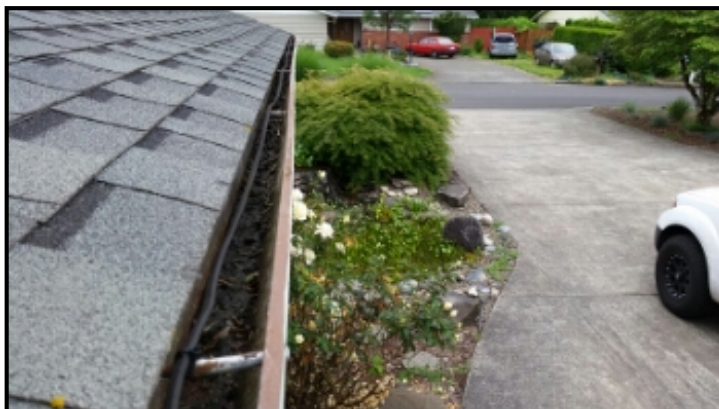
Gutter was used to run a coaxial cable. this adds additional strain to the gutter. recommend having the wires run in an alternate location.
