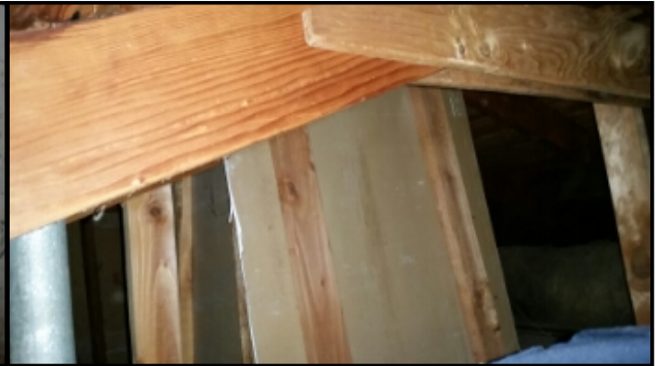
Sky lights are not insulated. this is a sizeable heat loss. Recommend having them insulated.
