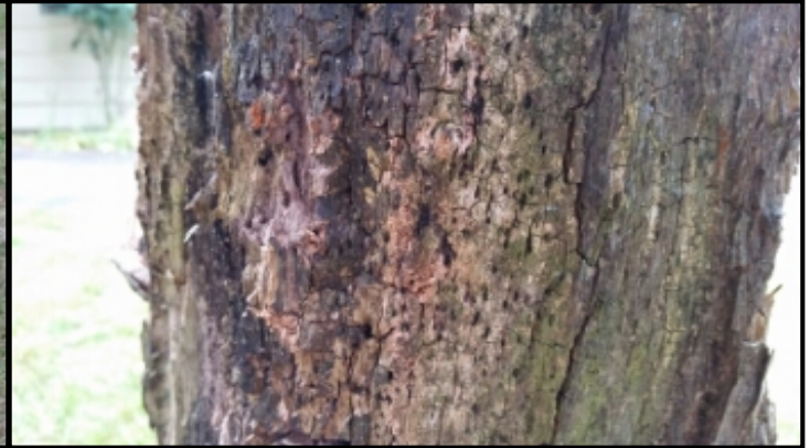
Possible exit holes in wood stump in back yard. Recommend removal.
