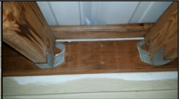
Shed roof attached to siding using framing nails. Recommend adding lag bolts for better dependability.
