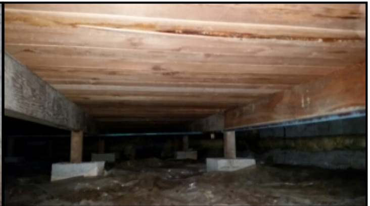
Post and beam construction. No floor insulation. Recommend insulating floor to avoid heat loss
