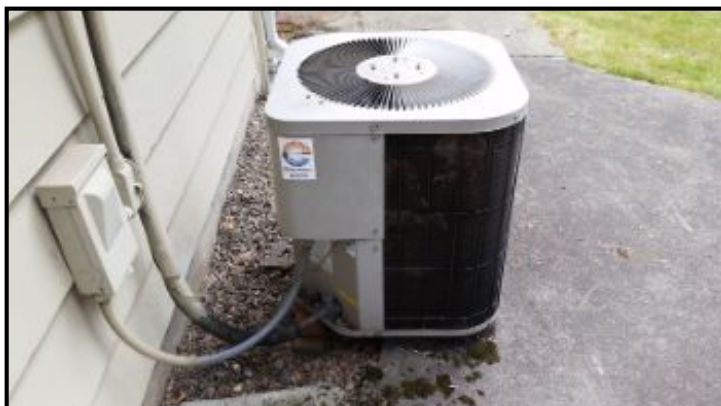
Air conditioner appears to be level, but it is not supported correctly. Only half of this unit is on solid ground. Recommend further inspection and support by a HVAC professional.
