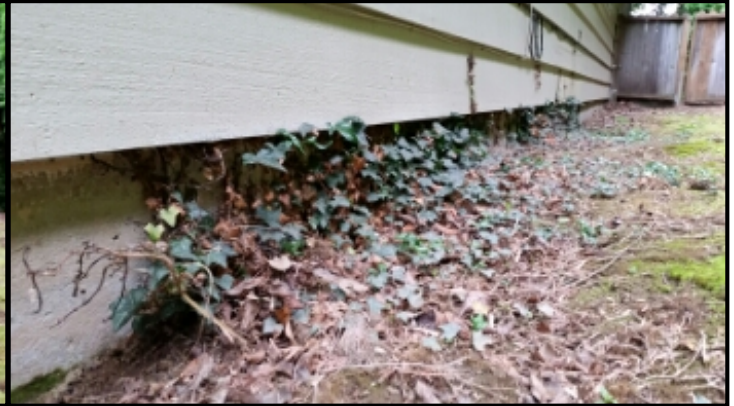
Ivy growing up foundation behind siding. Recommend removing ivy from foundation and monitor for reoccurrence. This is an invasive species.
