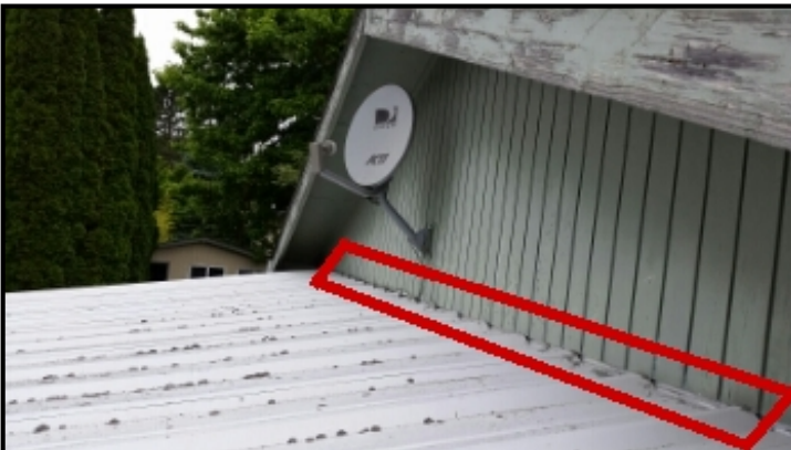
Shed roof flashing missing. This will invite rot. Recommend hiring a contractor to install in order to avoid water intrusion between ledger board and siding.
