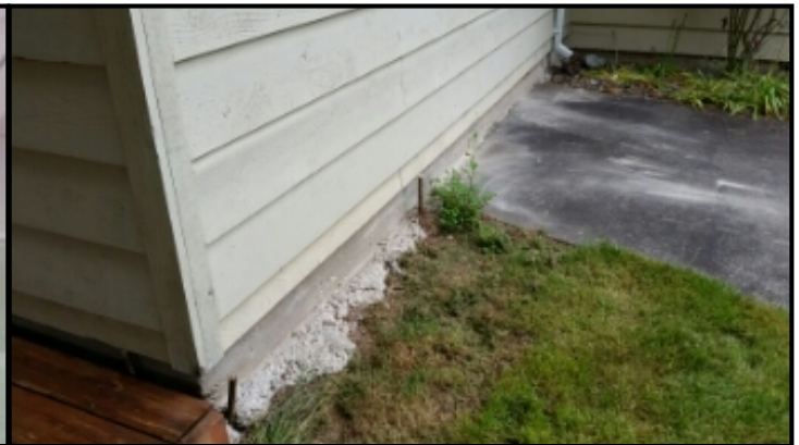
Addition in 2006 (per homeowner) is on a slab. Form holders never removed. this could be a trip hazard. Recommend removal.
