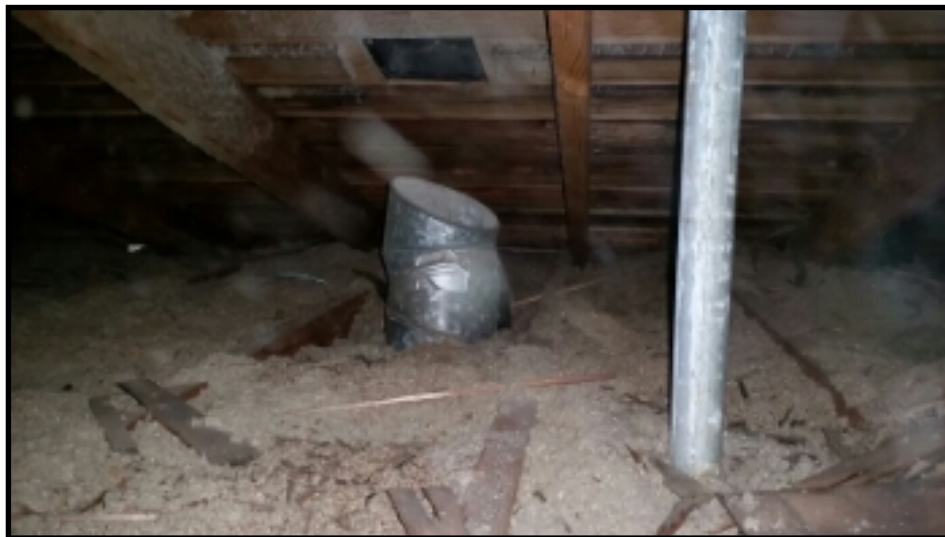
Master bathroom exhaust fan does not vent to exterior. Recommend having the duct run to vent outside attic space.
