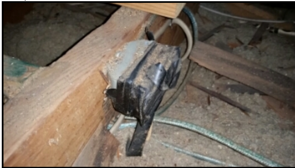
Improper cover over J box. Recommend having it repaired by electrician.
