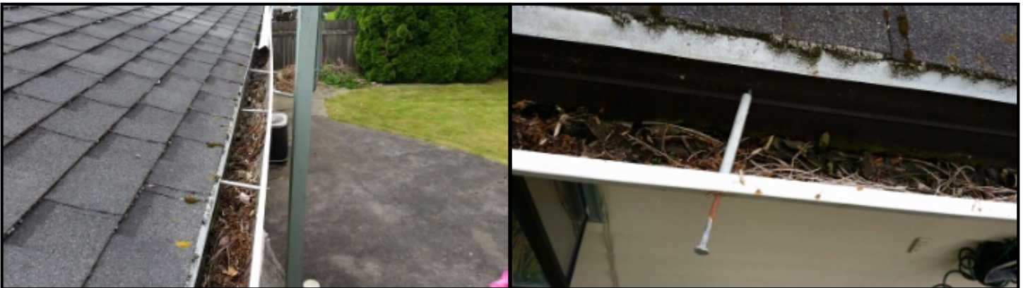
Gutter fasteners have pulled out of rafter tails. Recommend having them re-secured.
