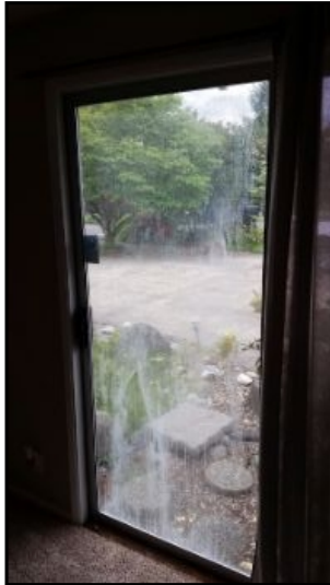
Duel glazed sliding glass door in master bedroom appears to have a broken seal. Recommend replacement.
