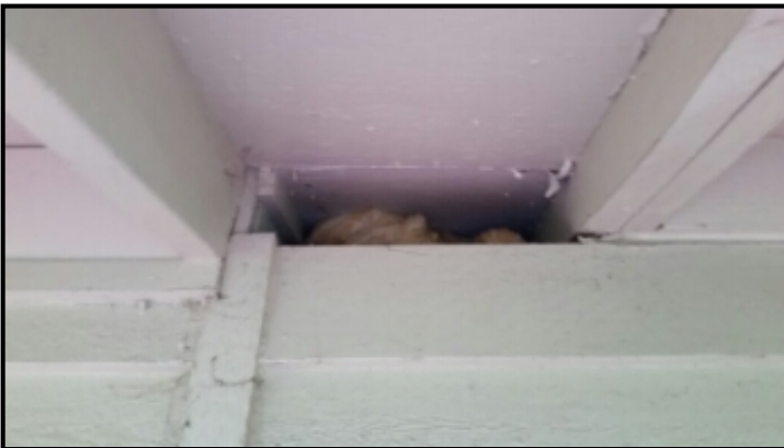
Soffit vent cover missing. Recommend replacement to avoid pests.
