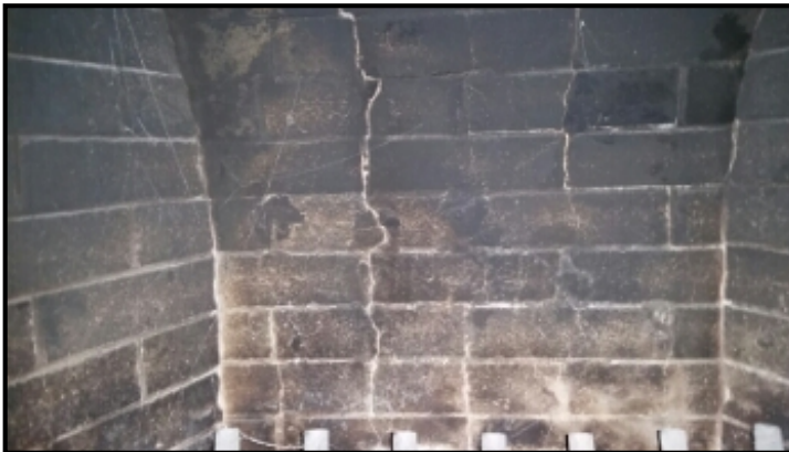
Fire bricks cracked/damaged; recommend evaluation by qualified technician.
