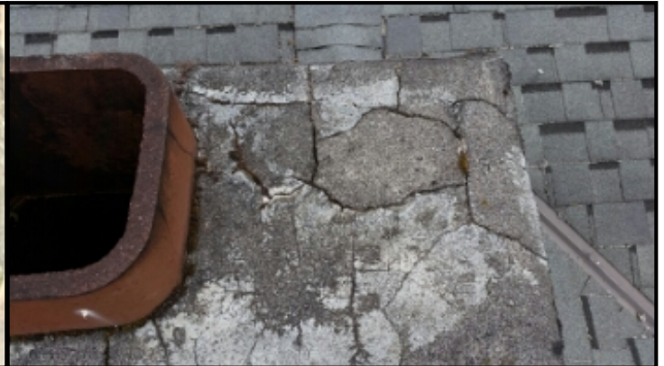
Chimney cap is failing. Recommend having a chimney expert review and repair if necessary.
