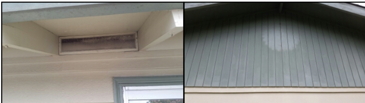
Eave vents blocked with insulation and paint overspray. recommend having insulation baffles installed and replacing the screens
