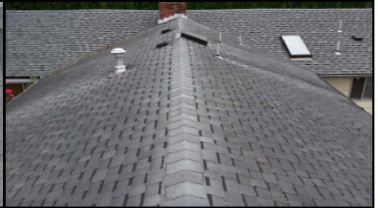
Roof covering appears in good serviceable condition.
