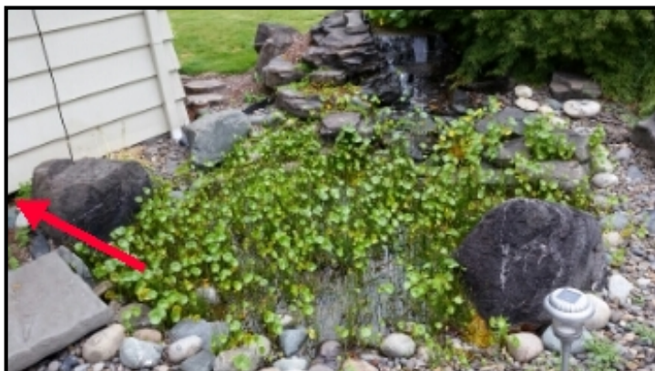
Water feature very close to the house. monitor water levels as to not allow it to overflow into the foundation vents (foundation vent marked with an arrow)
