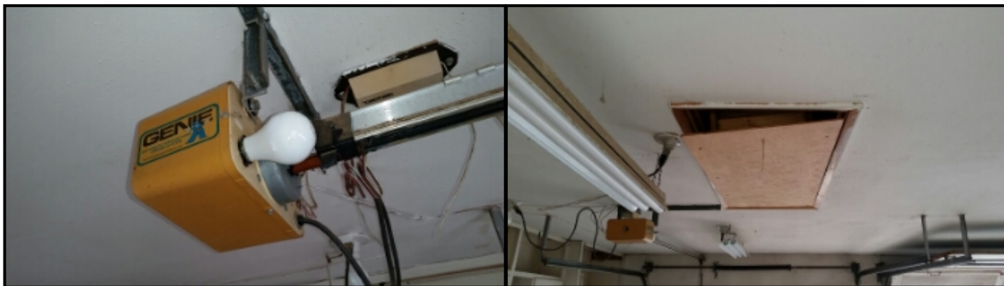
Garage door open failed reverse test. This is dangerous. Recommend replacement.
