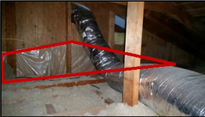
Duct to addition and uninsulated kneewall. Recommend having kneewall insulated to avoid heat loss.
