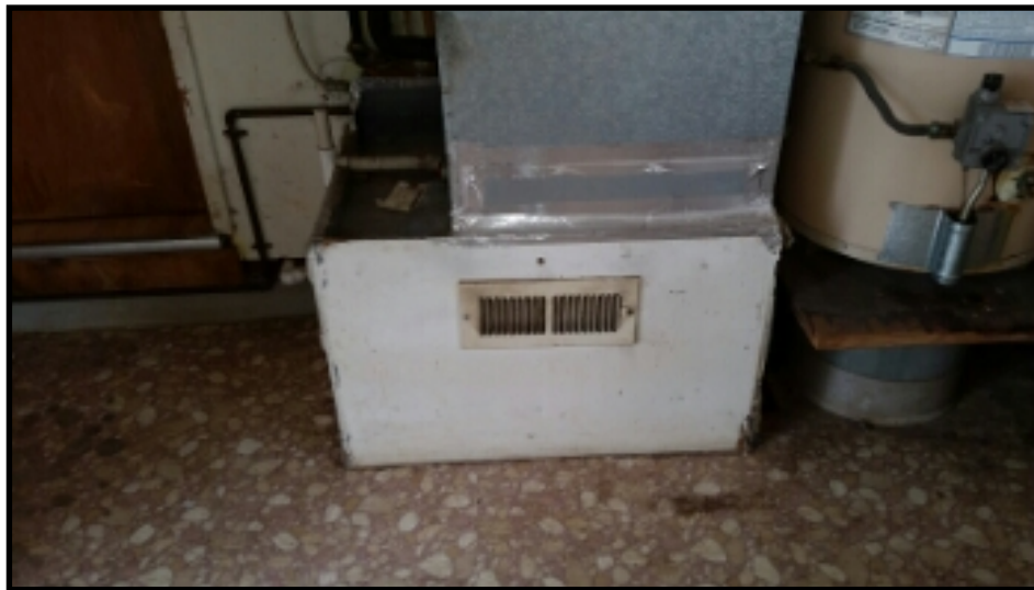
Plenum below furnace made of wood. This is not advised. recommend replacement with sheet metal by an HVAC technician
