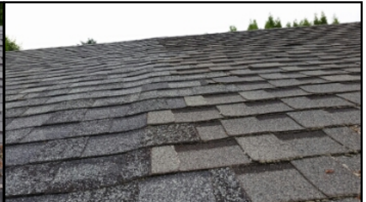
Roof covering change where addition roof meets older roof covering.
