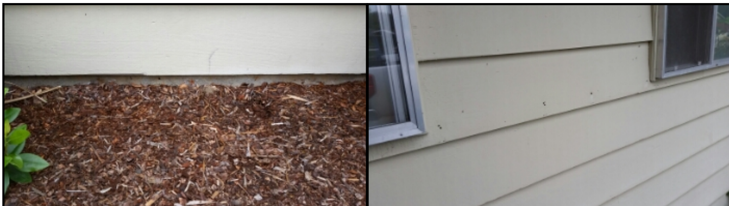
Siding-Soil contact or proximity. This may provide entrance of moisture or insects to siding. Recommend grading soil so there is at least 6" of space (where practical) between the siding and the soil below and checking for any damaged trim and siding materials. holes drilled in siding between bathroom windows. recommend patching and painting.
