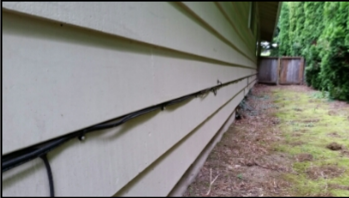
Wood lap siding. Good Condition.
