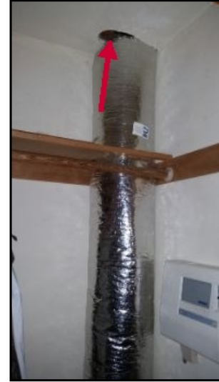
Supply duct to addition has an oversized hole and should be sealed to avoid heat loss and possible pest intrusion.
