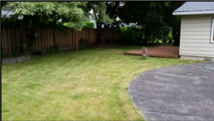
Grade appears flat, but lot is lower than rear bordering lot. monitor for water flow toward foundation from adjacent lot.
