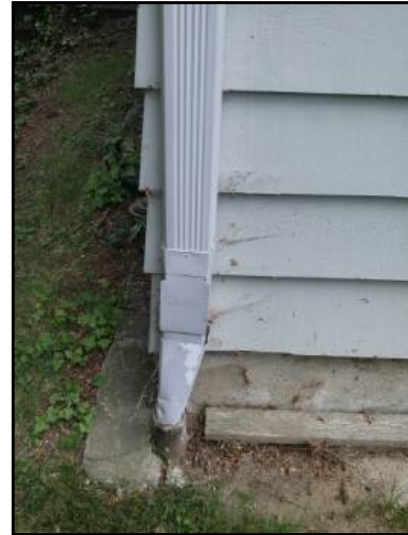
Most downspouts are attached to underground piping.
