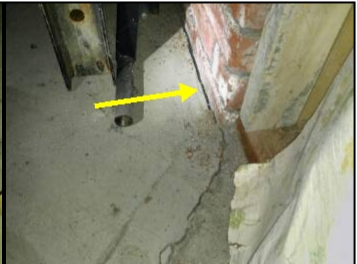
Cement slab is separating from chimney bricks
