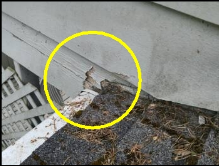
Exposed wood at gutters above deck
