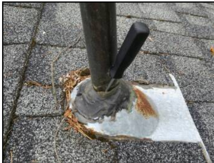
Flashing boots around plumbing vents are broken
