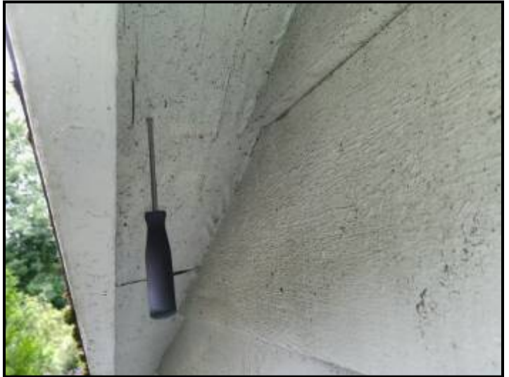
Roof decking is soft at edges under overhang
