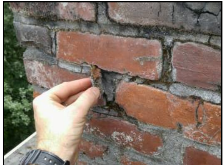
Mortar is cracked and broken around bricks.
