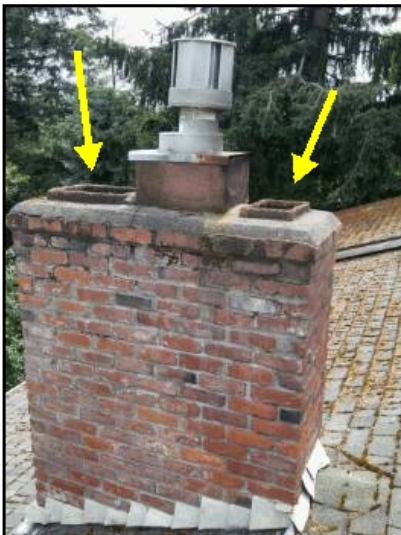
Spark arrestors missing
