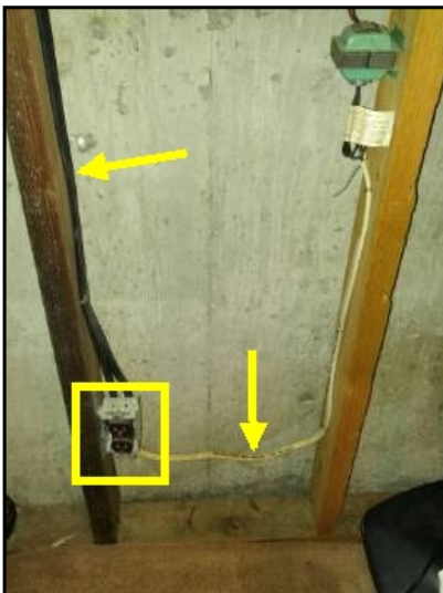
Out cover missing and romex wire not protected from accidental contact.
