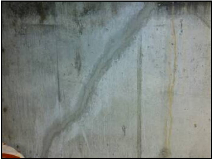
Foundation crack repair
