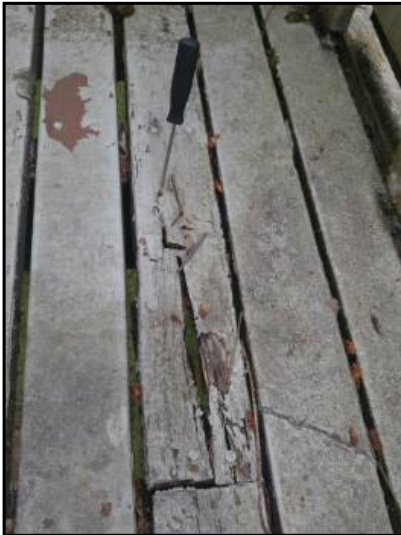
Wood rot observed on deck surface
