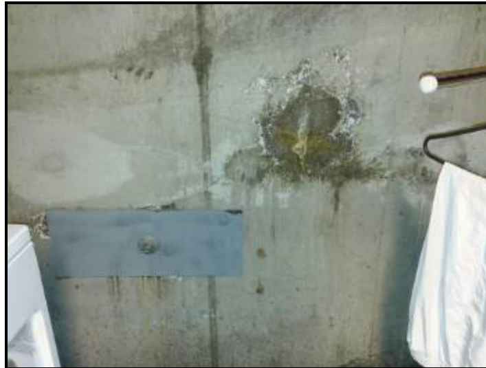
Horizontal crack in foundation was resupported. Repair appears to be done correctly
