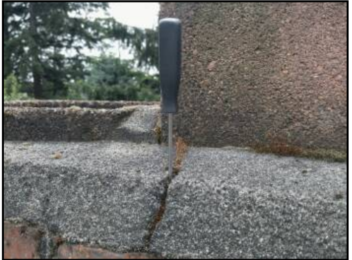
Chimney cap cracked and worn away at edges
