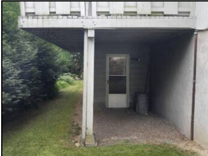
Support beam does not appear to be fastened to the pier pad below.
