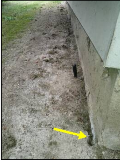
Potential pest tunnels at base of foundation. Soil is very hollow
