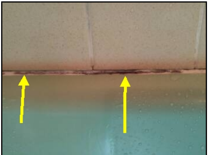
Black staining and breaks observed in bathtub caulking
