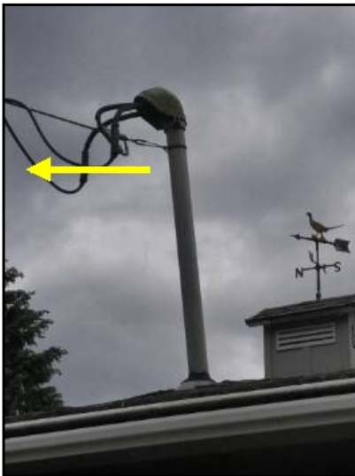
Electric service mast is bent
