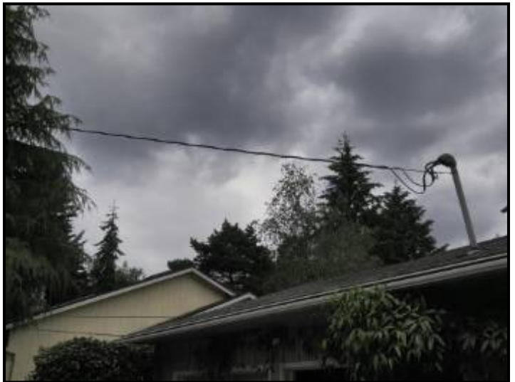
Electric service line has no slack.
