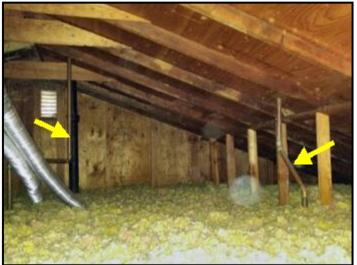
Copper venting pipes for plumbing system
