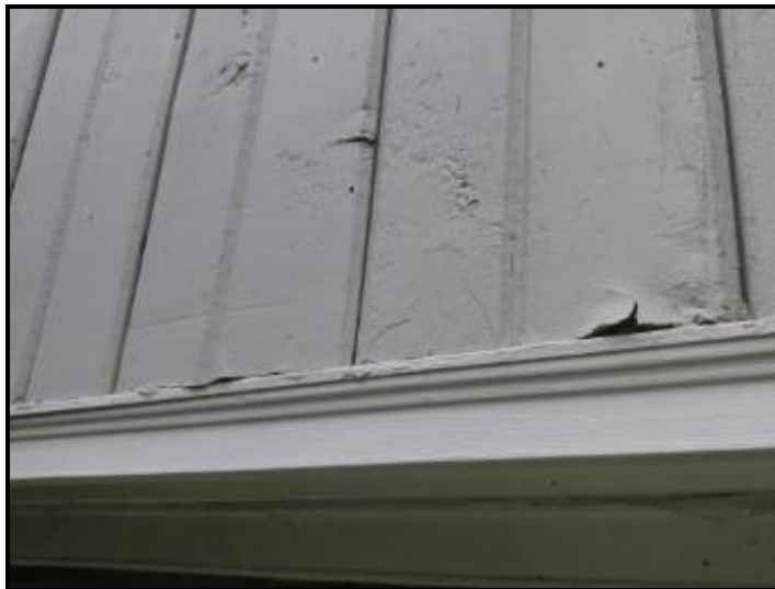
Siding paint peeling above window and door frames
