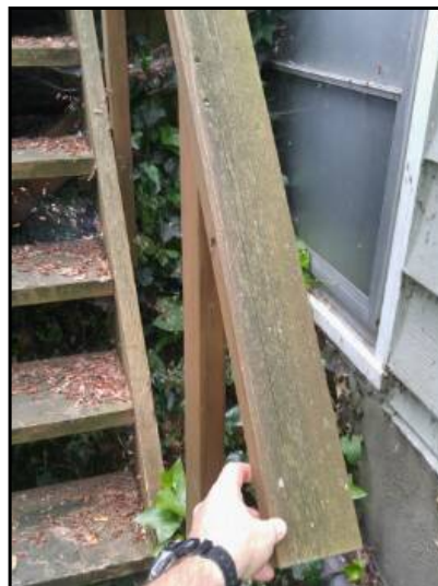
Handrail wobbly and only installed on one side. Safety concern
