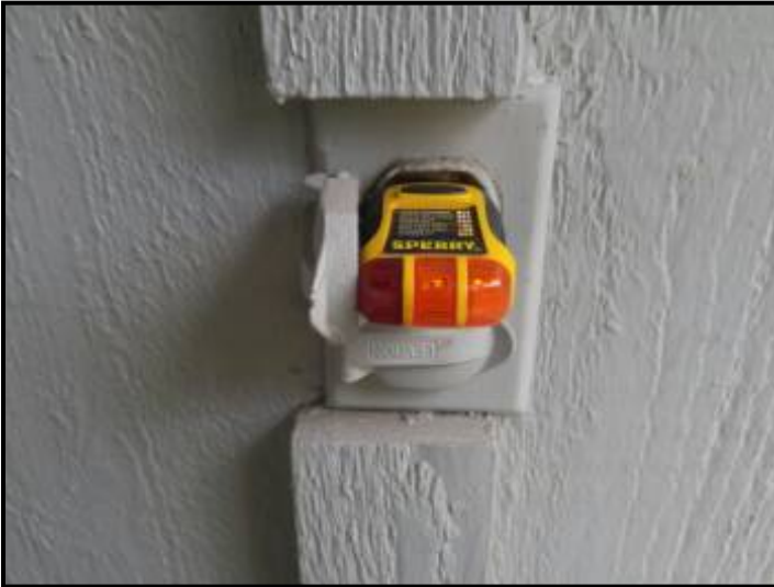
Exterior outlets are not GFCI Protected
