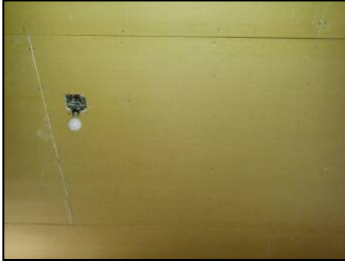
Drywall not finished in basement room
