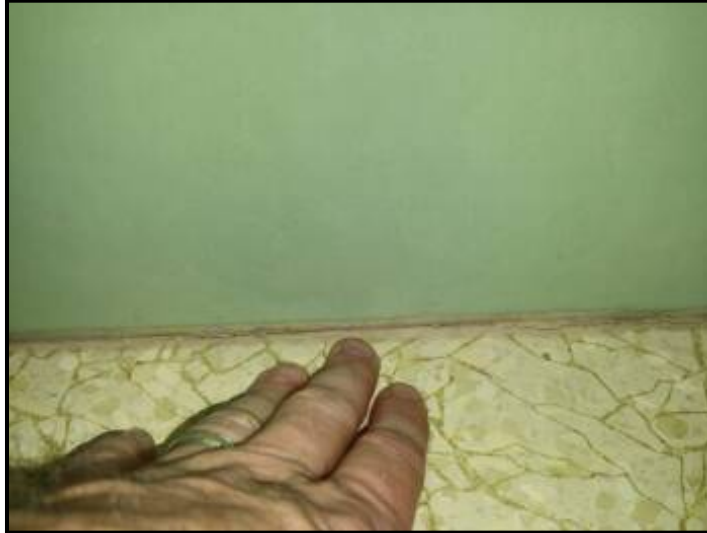
Caulking broken at tub/floor connection
