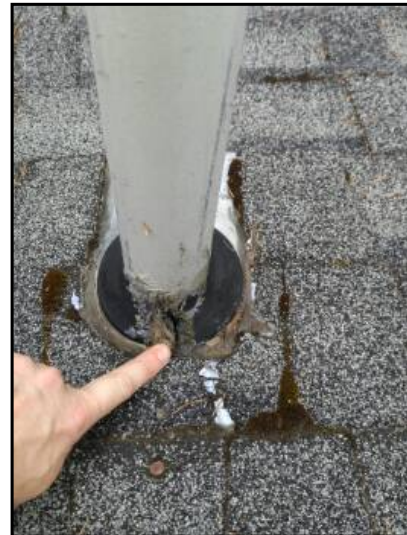
Flashing at base of electric mast is cut and sealant has failed
