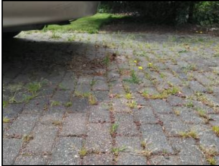
Sunken areas on brick driveway. Vegetation growth observed
