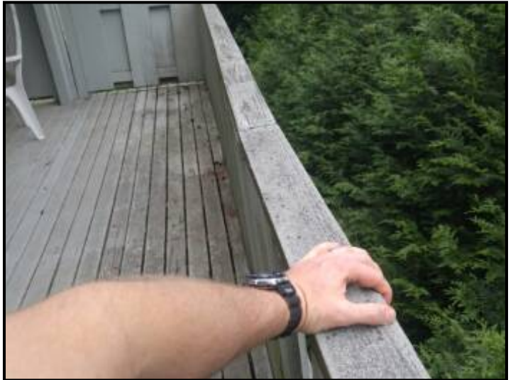
Railing is not secure
