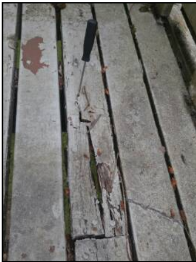
Wood rot observed on deck surface
