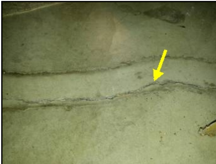
Large crack in basement floor appears to be recent. Repair made previously.
