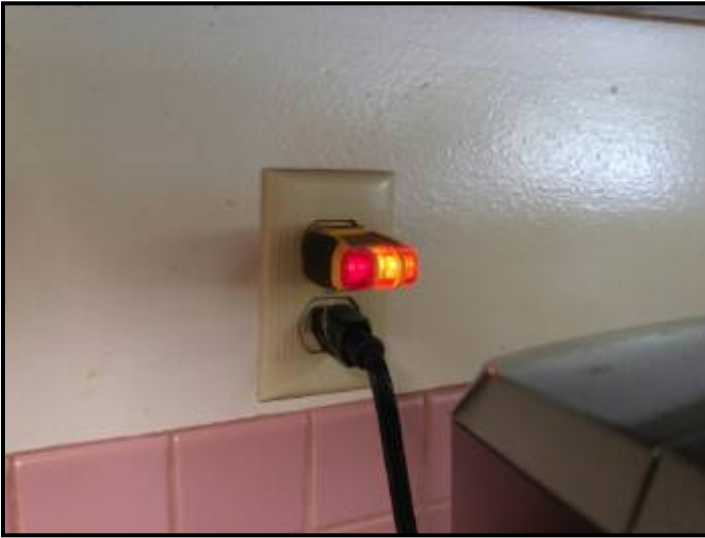
GFCI outlets not installed near water fixtures
