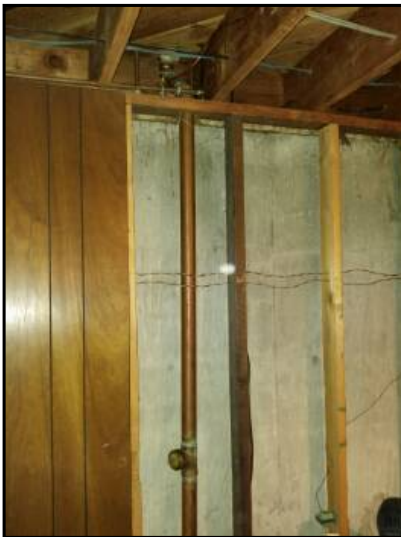
Waste plumbing is made of copper tubing.
