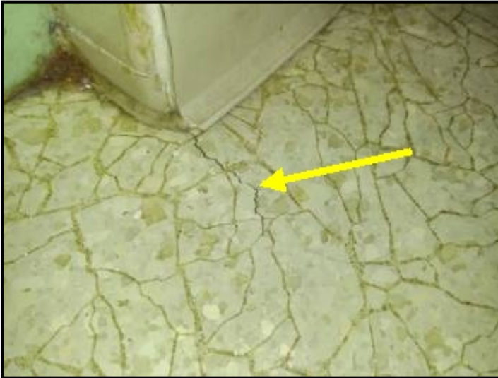
Crack in linoleum floor in bathroom.
