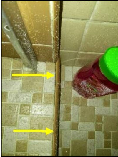
Tiles detached in master shower. Tile are loose to the touch
