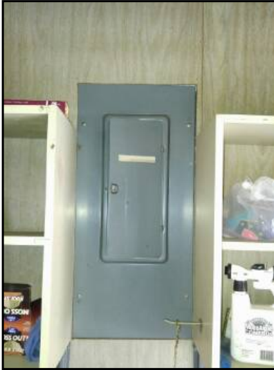
200 Amp Federal Pacific electric panel installed in garage
