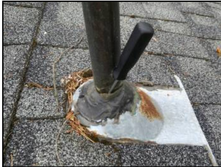
Flashing boots around plumbing vents are broken
