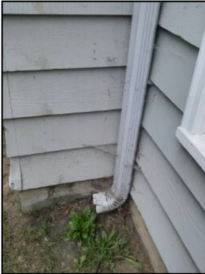
Downspout terminates at base of foundation
