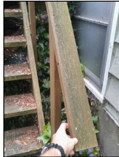
Handrail wobbly and only installed on one side. Safety concern
