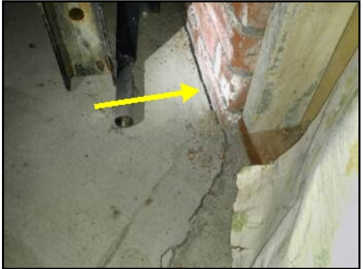
Cement slab is separating from chimney bricks
