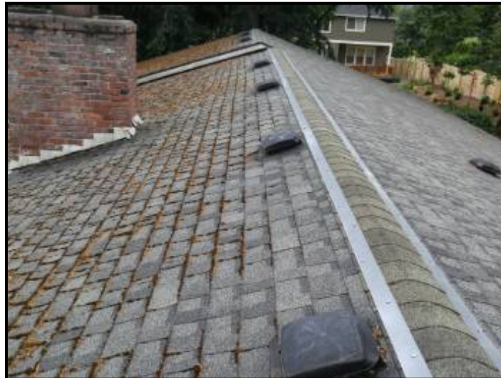
Upper attic ventilation installed
