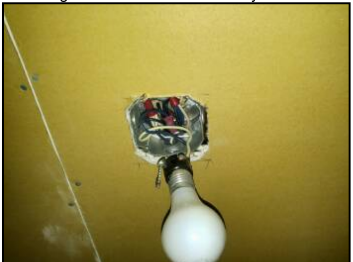
Junction box cover missing. Light fixture hanging by wires.
