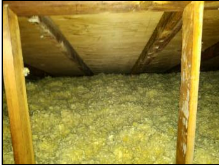
Loose fill blown in fiberglass. Ventilation baffles not installed
