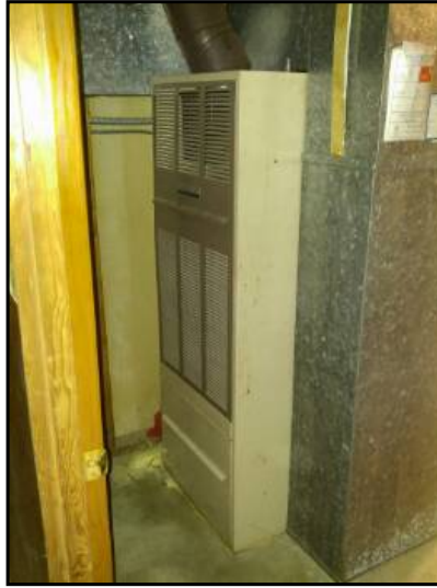
Oil furnace installed in basement
