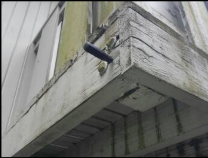
Wood rot at ends of support framing
