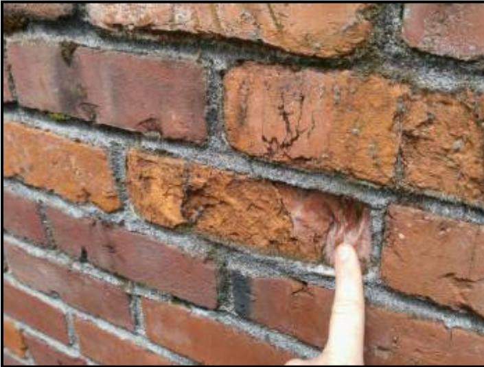
Bricks have spalling damage from freeze thaw cycles
