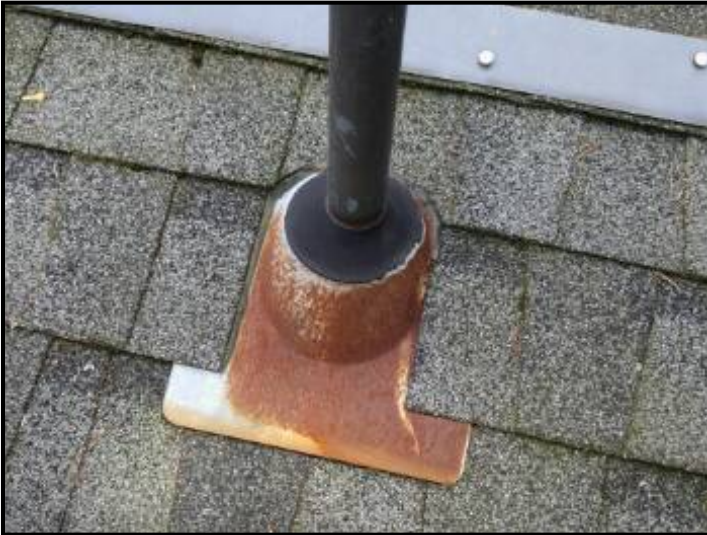
Flashing around plumbing vents is rusted
