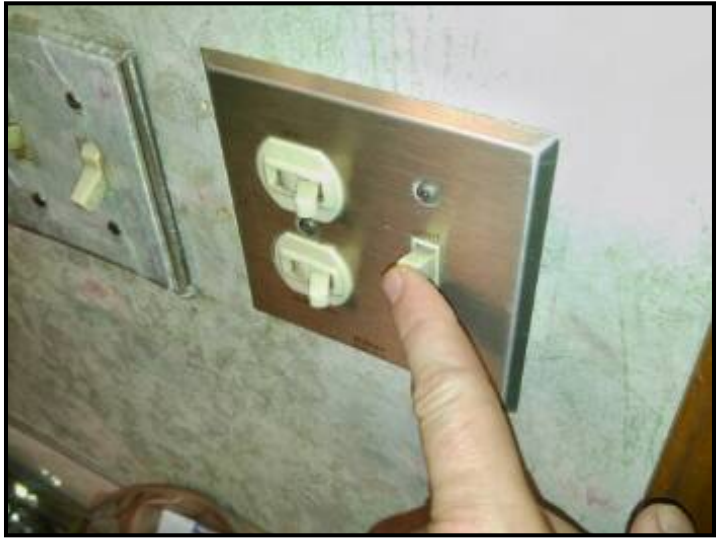
Light switch in hall bath is very loose.
