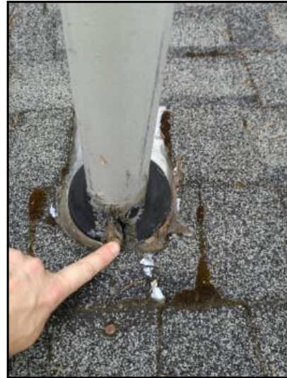
Flashing at base of electric mast is cut and sealant has failed
