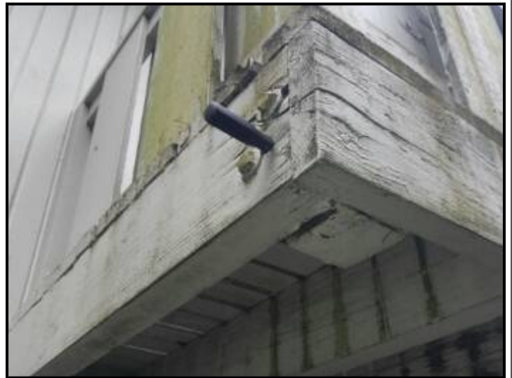
Wood rot at ends of support framing
