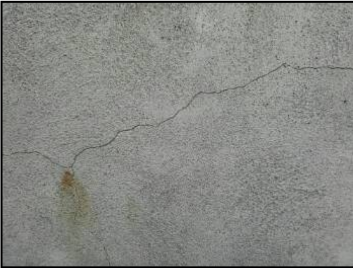
Foundation cracks observed
