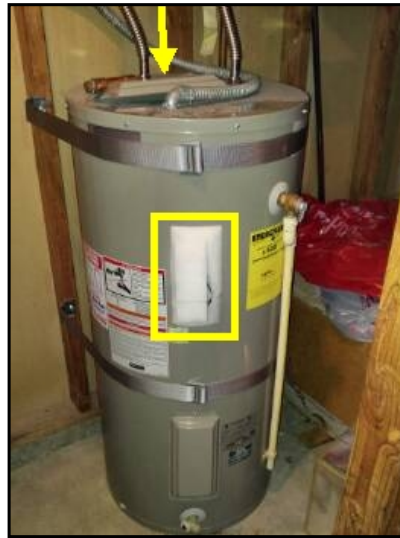
50 gallon electric water heater installed in basement in 2014
