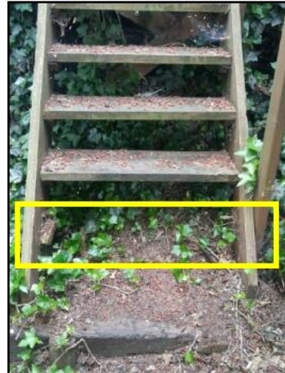
Step missing at exterior steps
