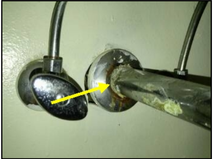
Corroded drain under master sink. Replace soon
