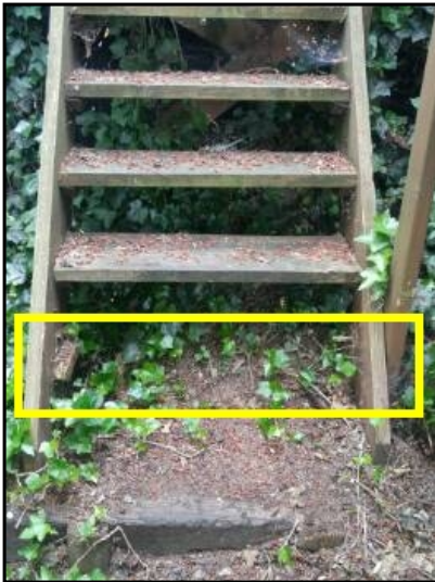
Step missing at exterior steps
