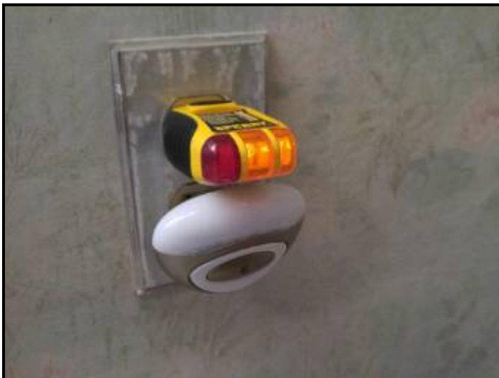
Outlets above sinks are not GFCI protected
