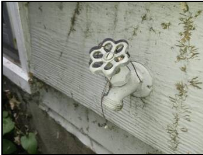
Exterior house bibs are shut off from interior at rear of house
