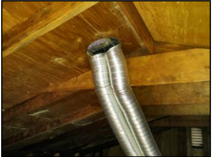
Upper bathroom vents vent toward a roof vent. A positive connection would be preferable.
